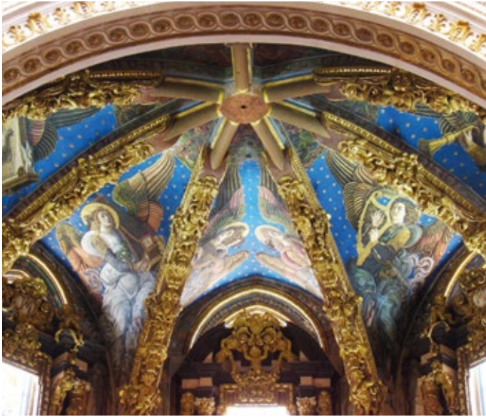
Figure 2. Detail of the dome. At the keystone, only the ends of Gothic arches are visible; the remaining parts are covered with Baroque decoration. Between these Gothic/Baroque arches, the Gothic ceiling is covered by Renaissance paintings. In order to make the Renaissance paintings fully visible, the massive hanging Baroque keystone was removed. What can now be seen is a blank, octagonal one.
